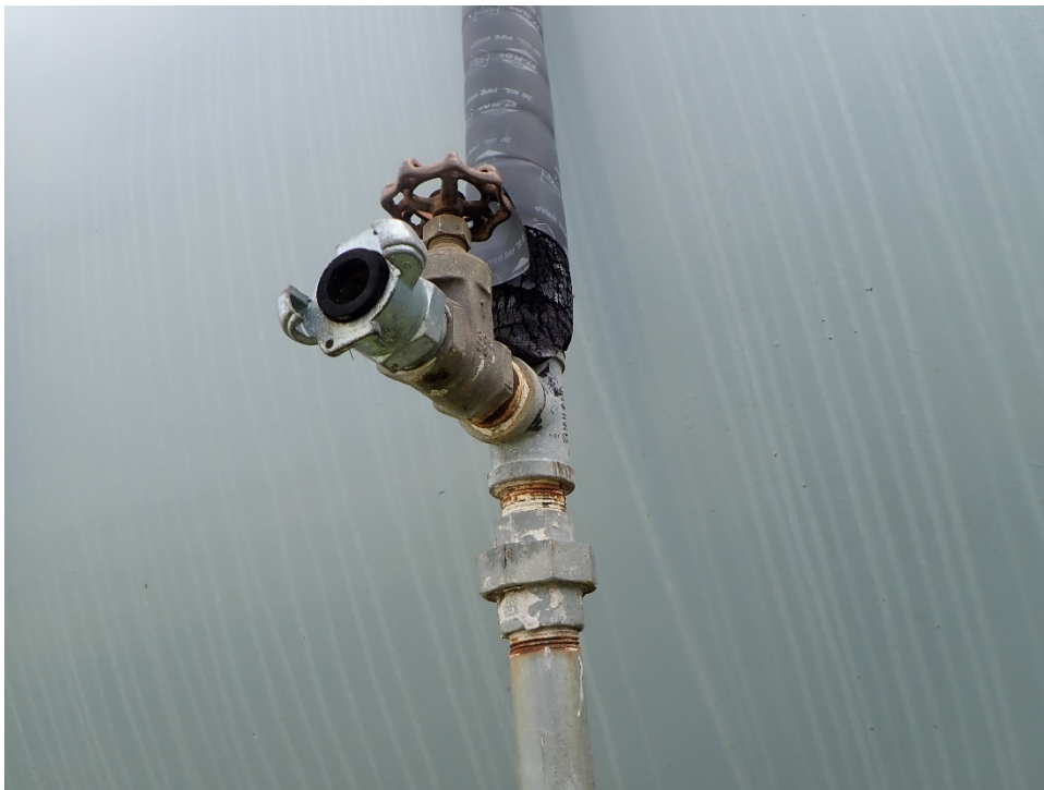
Photo 4: Crows foot and air line with corrosion
