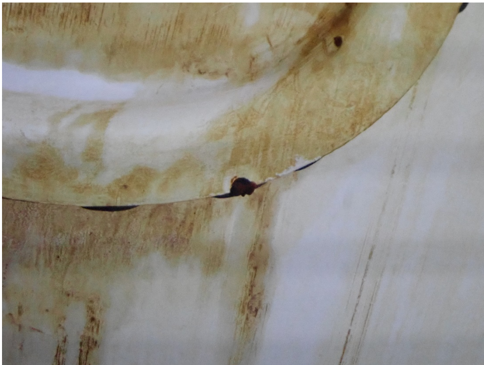
Photo 8: Interior elliptical hatch with corrosion
