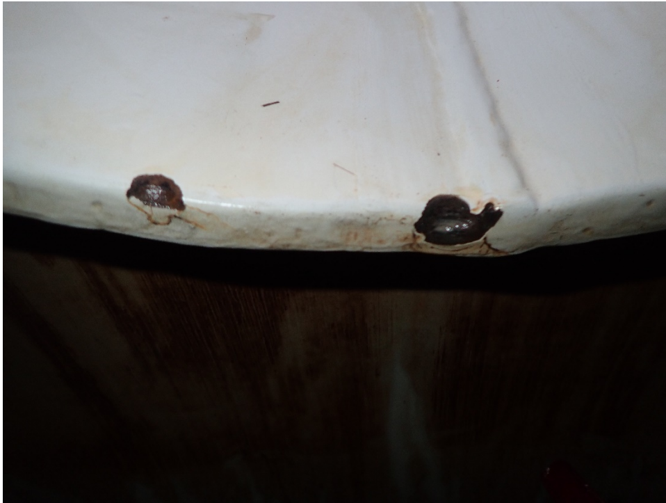
Photo 7: Interior manway edge with corrosion
