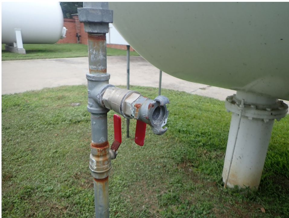
Photo 2: Crows foot and air piping with corrosion
