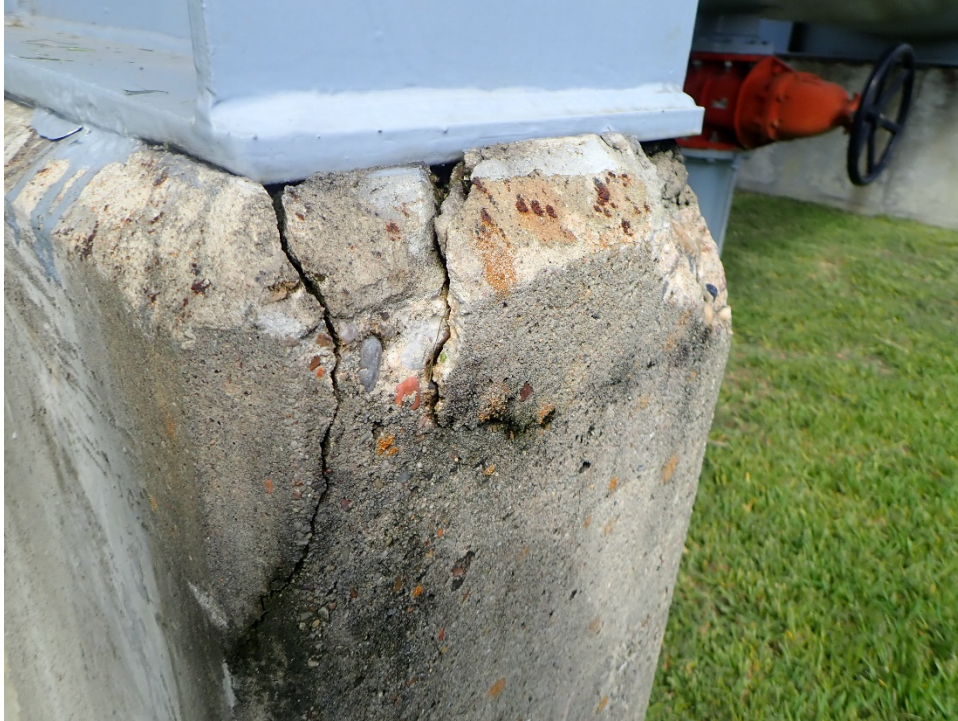
Photo 1: Concrete tank footing with spalling
