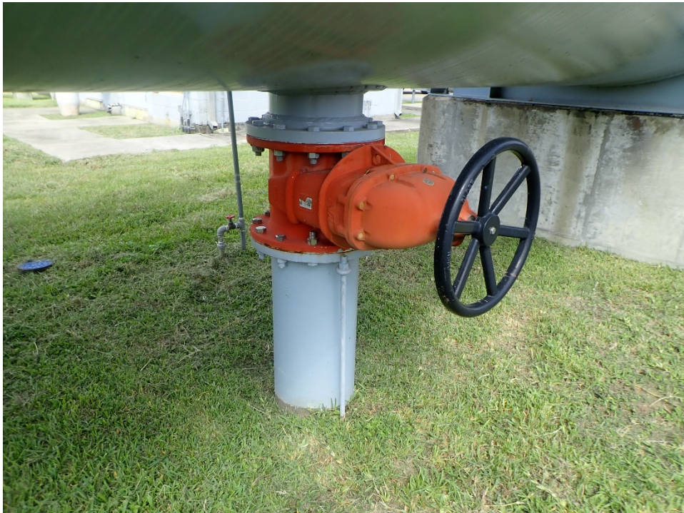
Photo 2: Inlet/outlet line with corrosion
