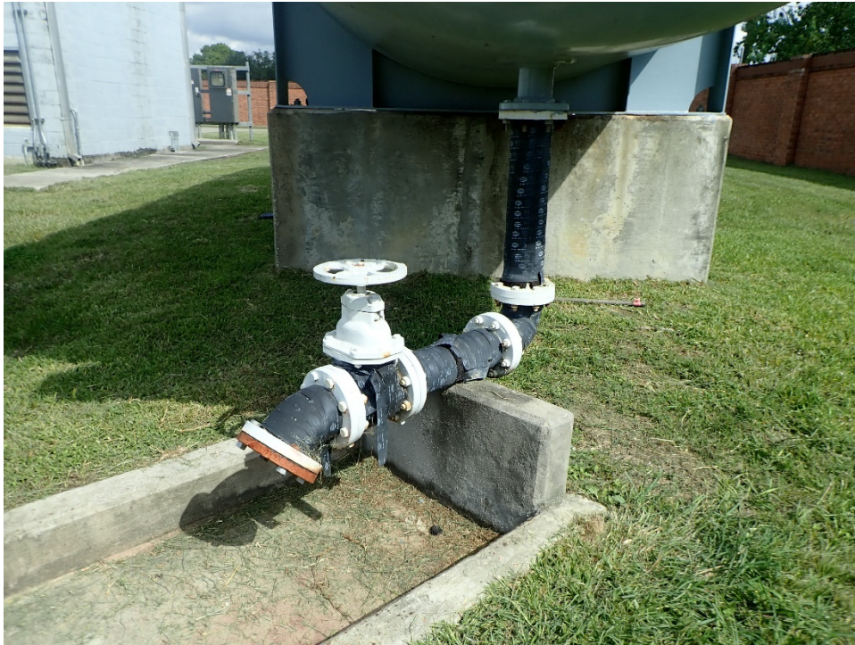
Photo 3: Drain line with corrosion
