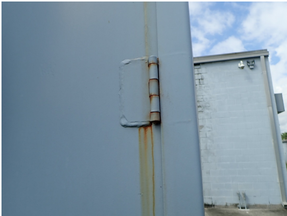
Photo 6: Equipment box with rust bleed at hinges
