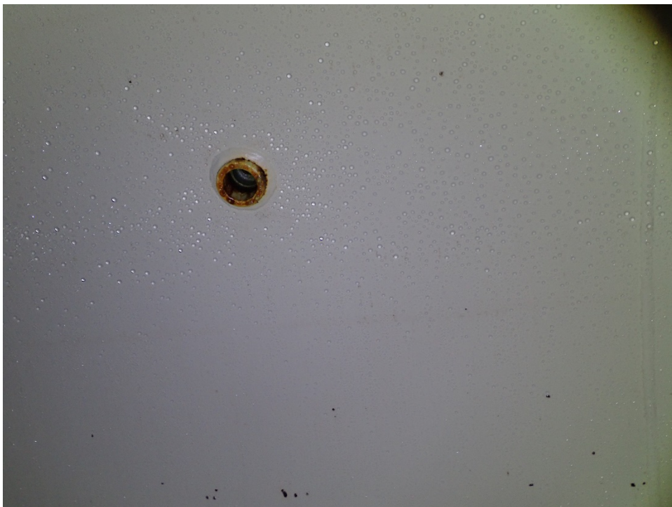
Photo 6: Interior penetration with corrosion
