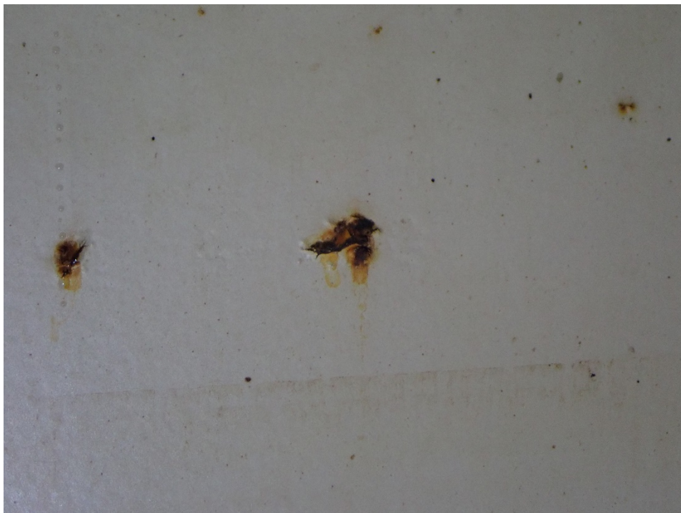
Photo 4: Interior walls with corrosion
