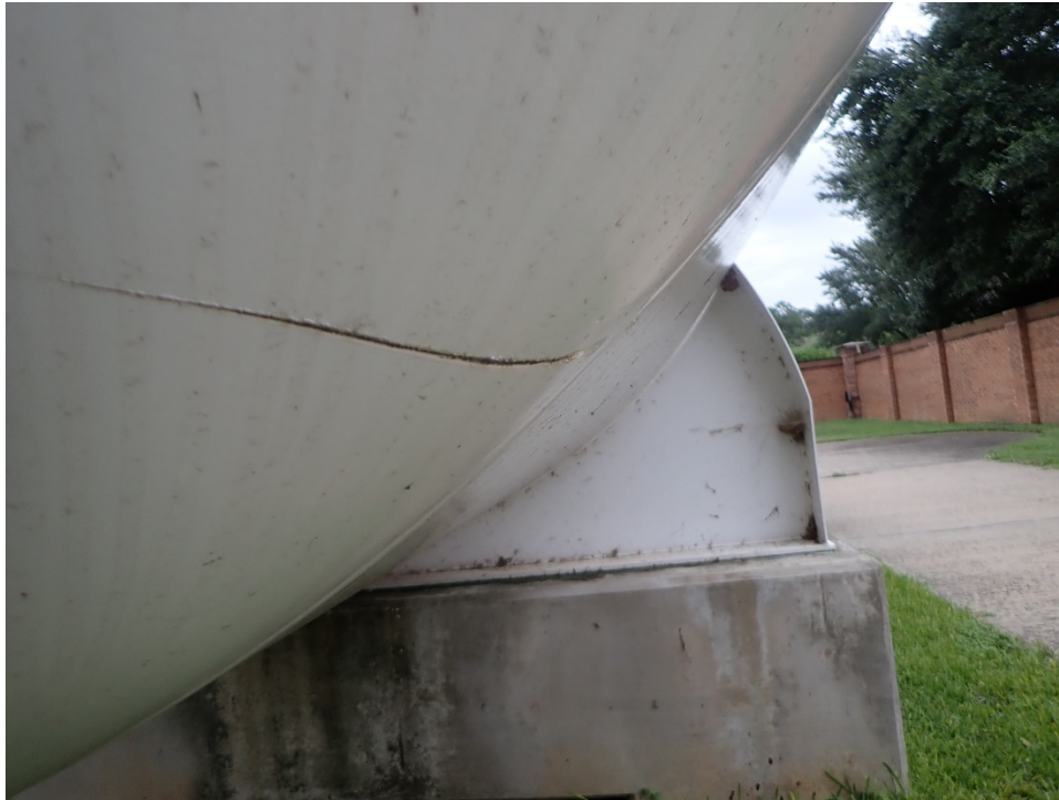
Photo 1: End cap with a scratch and corrosion
