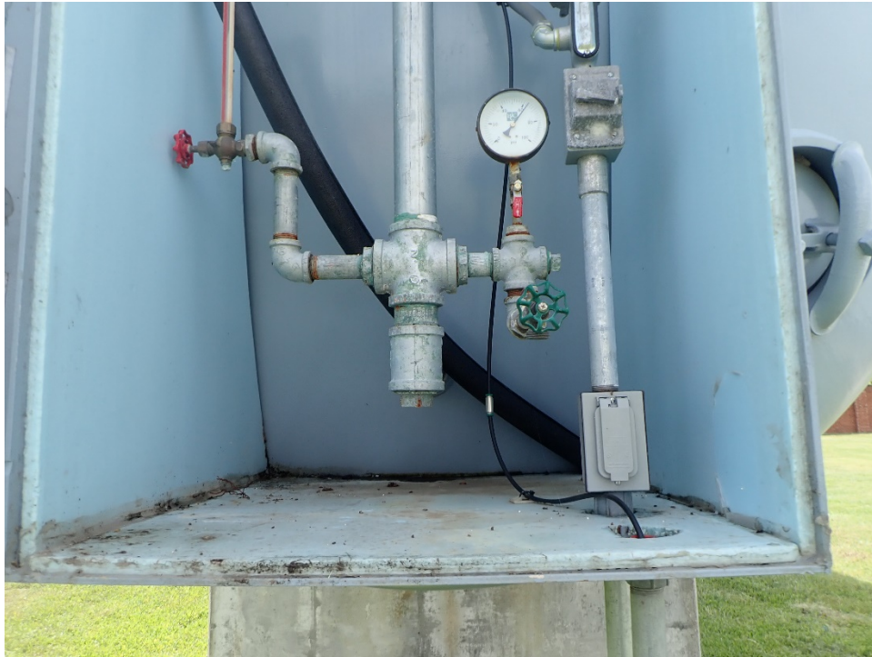
Photo 5: Equipment box piping with corrosion
